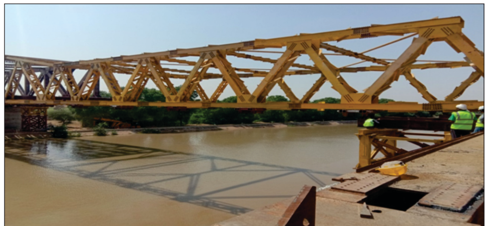
Fig. 2 : Photograph During Launching of Truss
