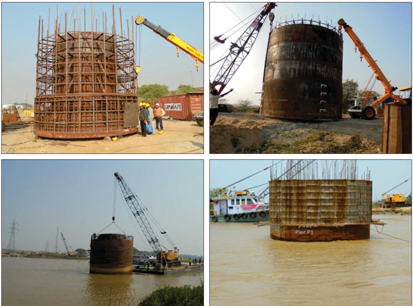
Fig. 2 : Floating Caisson and Casting of Steining
