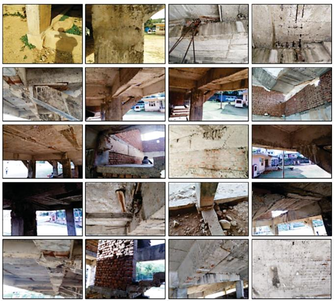
Fig. 3: Signs of deterioration
