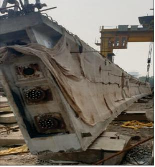
Photo 2: Plan Bending after shifting of girder from Casting Yard
