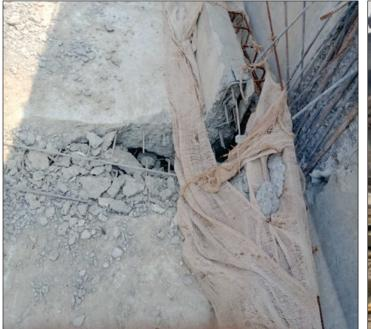
Photo 1: Girder Break at 3L/8 Location during Lifting
