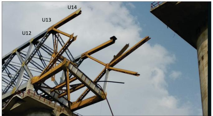
Fig. 6: The snapped anchor span - the snapping joint at U14 shows no full-strength splice
