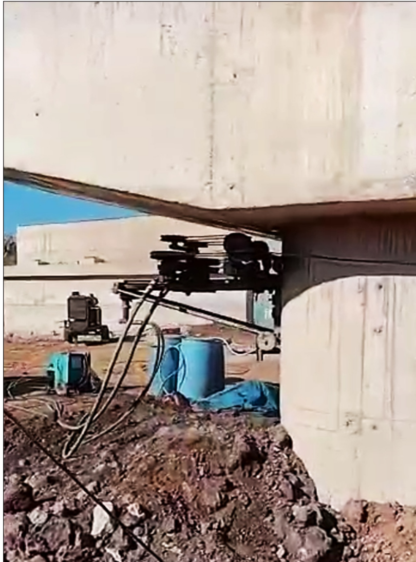
Fig. 6 : Image showing pier being horizontally cut by diamond cutting.
