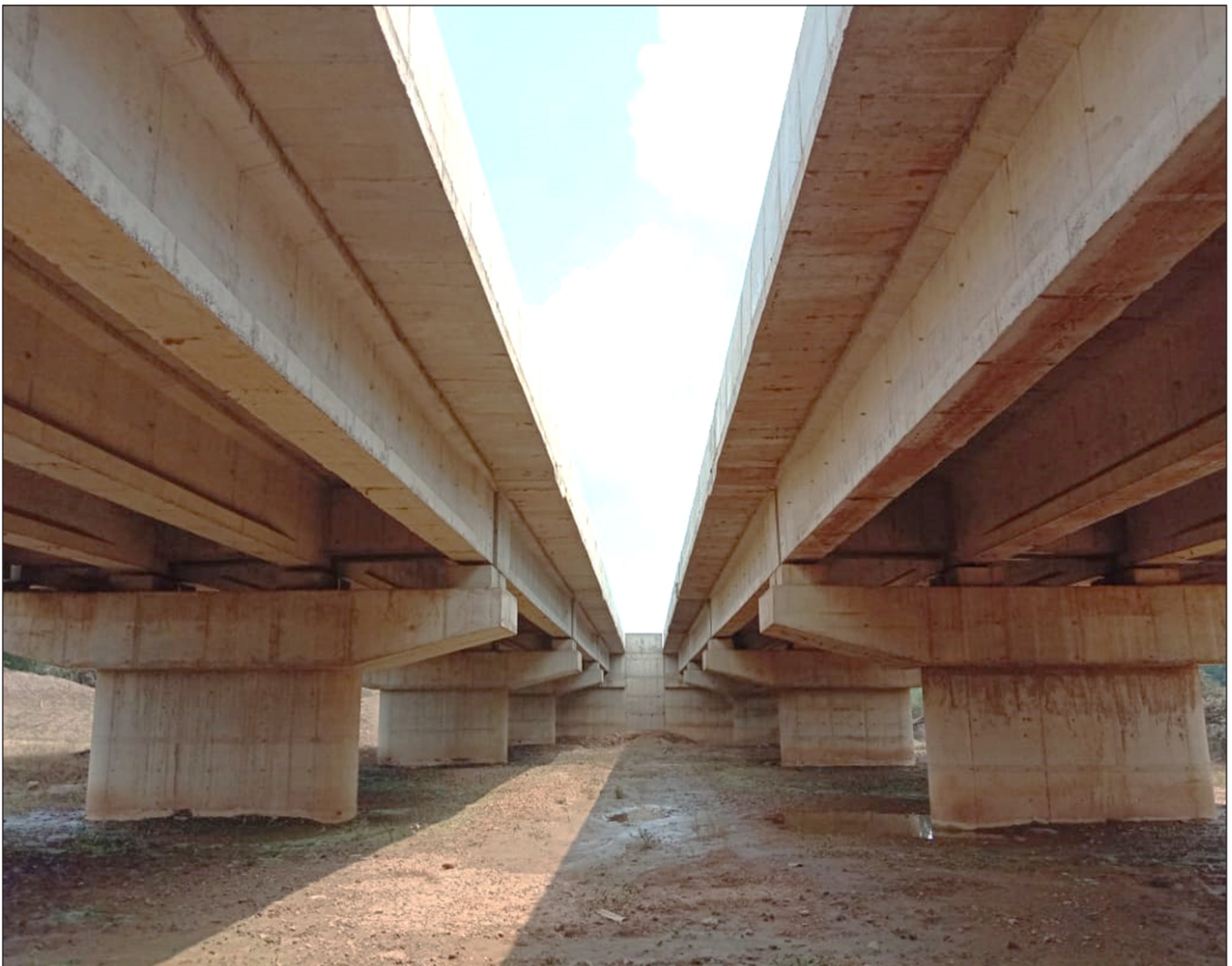
Fig. 1 : Major Bridge on NH passing through rural central India
