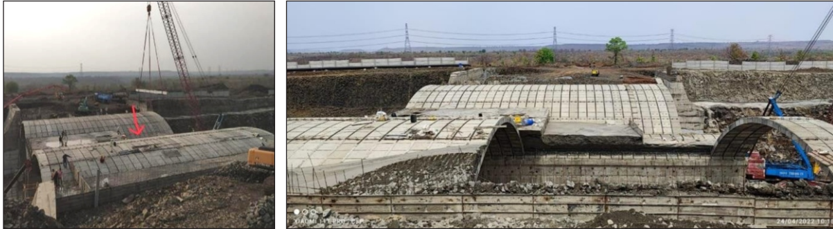
Fig. 4 : Photo just before and after collapse
